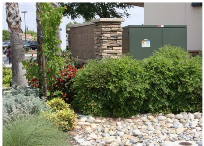
Utility Box Example
