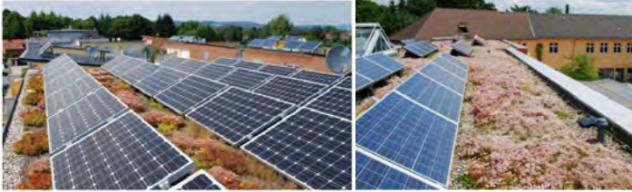
Figure 4.17: Case Study: Solar Panels and Green Roofs Fully Integrated - Breuning, Tilson
