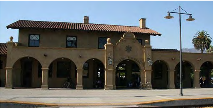
Figure 2. 24: City of Santa Barbara Train Station in Mission Revival Style
