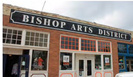
Figure 1.18: Example of an arts district in an adaptive reused warehouse structure in Dallas, Texas
