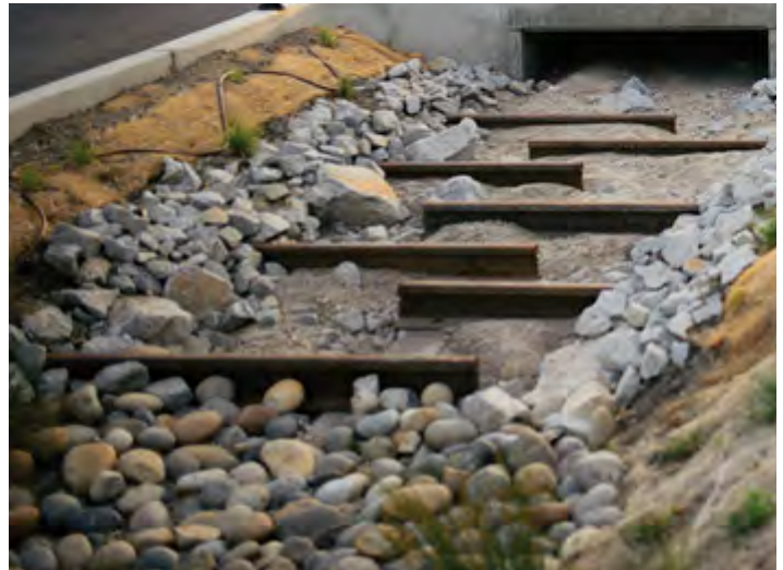
Figure 3.7: Bioswales in Paso Robles The City of Paso Robles implemented bioswales along 21st Street to mitigate flooding that often occurred during heavy rains. The implemented design also helps to recharge the groundwater sources and prevents damage to street surfaces and buildings by preventing flooding.
