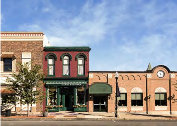
Figure 1.3: Maintaining the scale and facades of a small-town, this streetscape is engaging, varied and attractive.
