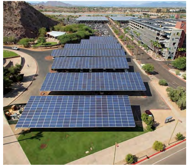
Figure 4.16: Case Study: Arizona State University. Solar parking canopies provide shading and an opportunity to generate energy.
