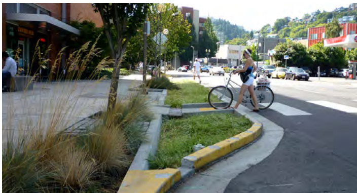
Figure 1.12: Well-designed crosswalk for pedestrians and cyclists alike, plus ample landscaping and bulb-outs as a traffic calming measure (Hoboken, NJ)
